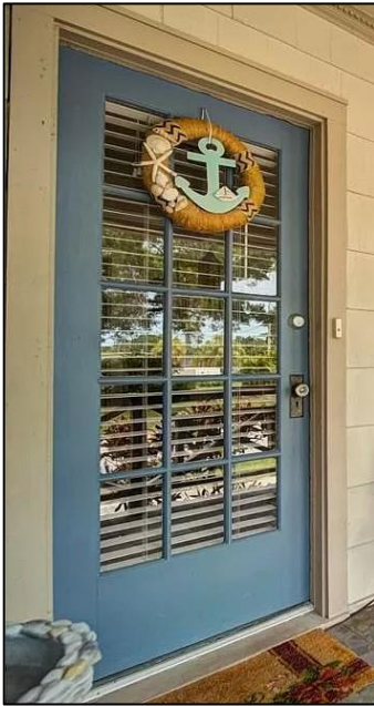
Figure 1: Door prior to replacement. Image from Zillow listing from the summer of 2020.
